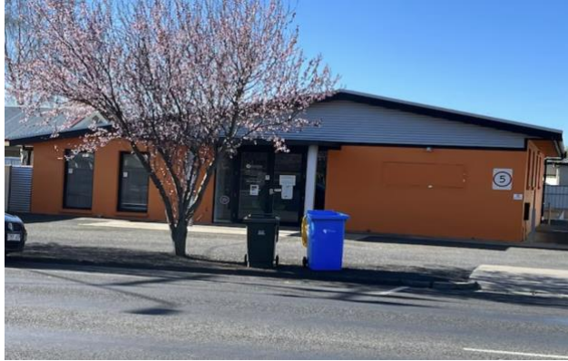
Image of the rehabilitation building (Eugene Boisvert & Sam Bradbrook, 2023) Screenshot (H)
